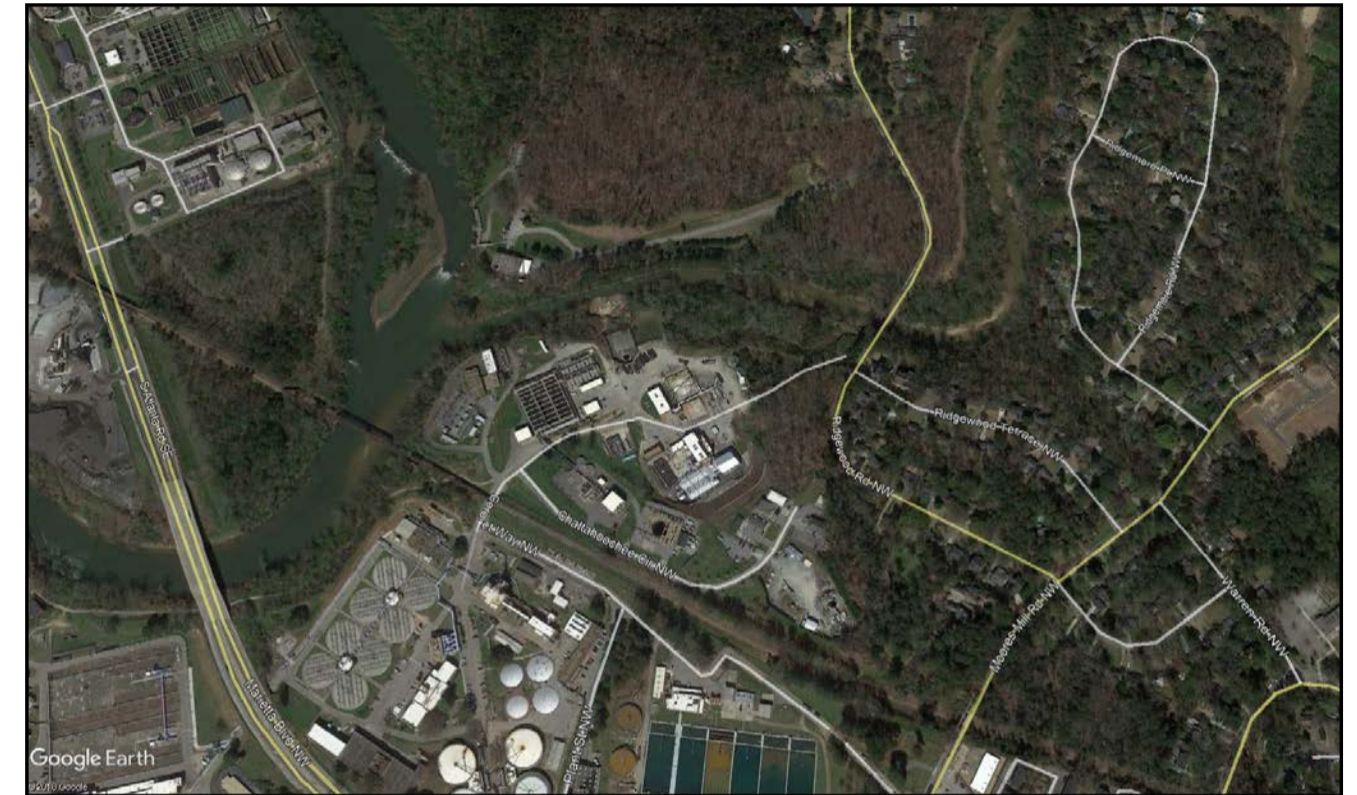
RIVER INTAKE PUMP STATION NTS 2630 RIDGEWOOD ROAD NW ATLANTA, GA 30318 FULTON COUNTY
