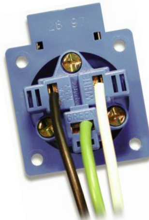
Wiring of Receptacles
